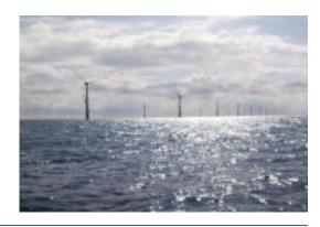
Northwind owns and operates an offshore wind farm located in the Belgian EEZ (exclusive economic zone), 37 km off the Belgian coast. The wind farm consists of 72 Vestas V112 3MW wind turbines with a total capacity of 216 MW.
