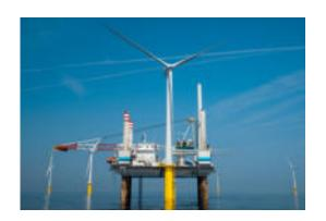
Nobelwind owns and operates an offshore wind farm 46 km off the Belgian coast. The wind farm consists of 50 MHI Vestas V112 3,3 MW wind turbines with a total capacity of 165 MW.
