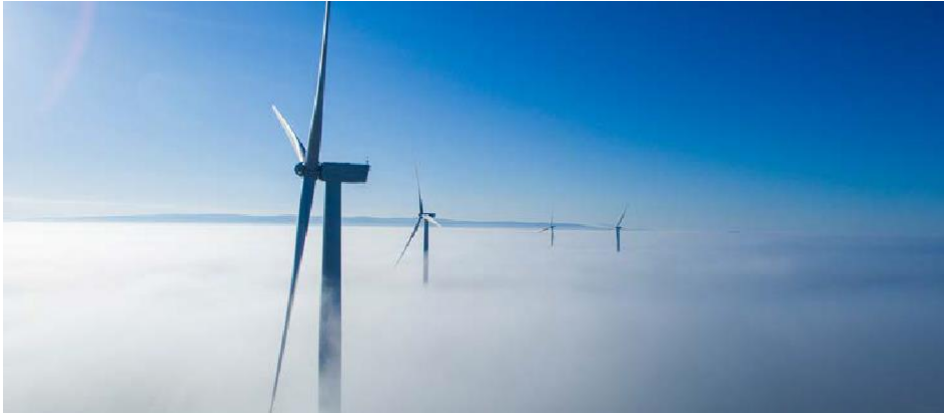
Storm Wind Ireland is an onshore windfarm in County Offaly, Ireland. The windfarm consists of 4 turbines with a total capacity of approximately 11MW.
